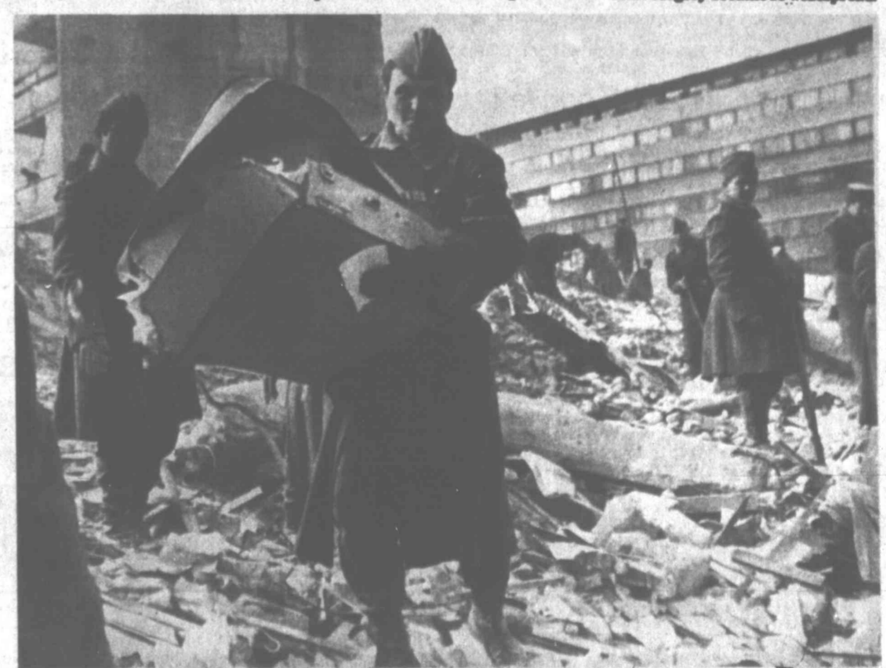
RESCUED FROM RUINS — A Romanian soldier carries a battered suitcase of belongings from ruins of a collapsed building Sunday. Soldiers and other rescue workers are probing rubble of buildings shattered by an earthquake that struck two days ago. More survivors were pulled from ruins Sunday but the death toll, officially placed at more than 600 persons, was expected to rise above 4,000.
