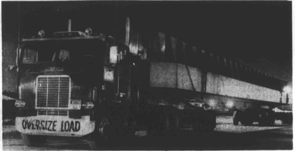
MONSTER RIG — This 36-wheeled monster, weighing almost 100 tons fully loaded, stopped in West Memphis Monday night on its 2,700-mile trip from Seattle, Wash. to Hollywood, Ala. The truck and load, which requires drivers front and back, is 130 feet long and 10 feet wide. The load can only move during daylight hours because of its size. (AP WIREPHOTO)
