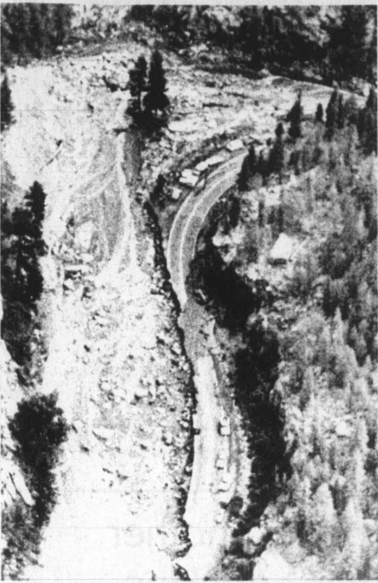
SLICED ROADWAY — Motor vehicles are backed up and stranded Sunday on either side of a slice knocked by flood waters from U.S. 34 through the Big Thompson Canyon. The river rushes by on the left.
