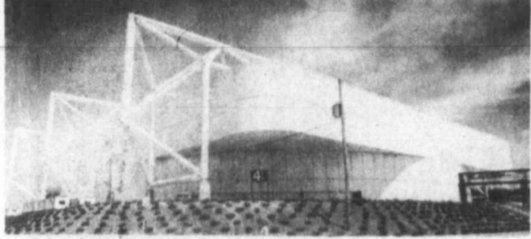
GLISTENING IN THE SUN — Kansas City's Kemper Arena will house the 1976 National GOP convention in August. Built to accommodate Kansas City's hockey and basketball teams, the arena's ice floor has been removed to make room for the convention.
