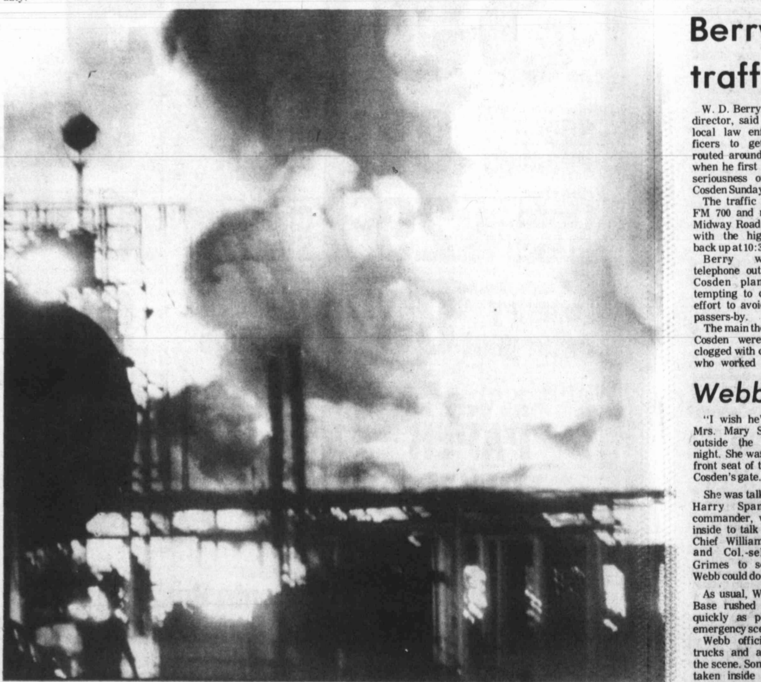
THE HEAT — Only fire fighters and Cosden officials knew the full intensity of the heat from Sunday's blaze, but the photograph by Herald Chief Photographer Danny Valdes gives some ideas.
