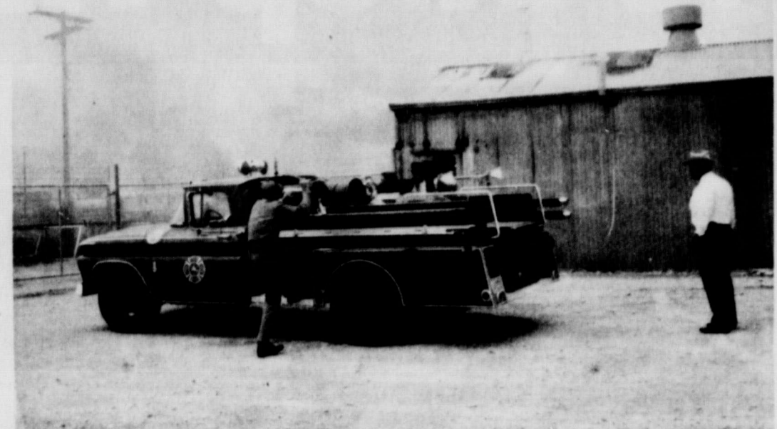
The Spearman Fire Department answered a call at noon Monday when the J.M. Huber office building, located just across the tracks from the Santa Fe building, downtown Spearman was heavily damaged by fire. Cause of the fire was unknown.
