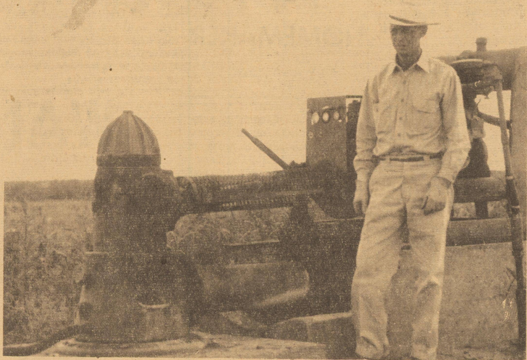
SAFETY--Roy Dodson displays one of the safety precautions on his farm west of Bovina. The open irrigation pump shaft can cause serious injury or even deaths if it catches loose clothing. The wire shield keeps clothing from being caught in the shaft.
