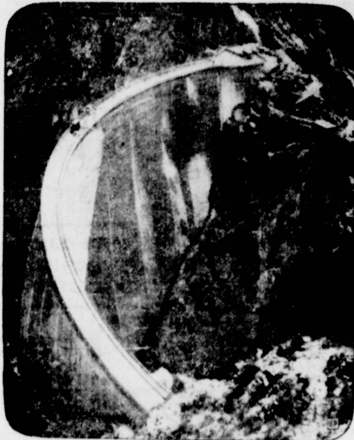
An interesting view of the Pacoima Dam at San Francisco, Cal., which has just been completed at a cost of $2,500,000. It was built by Los Angeles county as part of its water conservation program and drains 23 sq. miles in the Sierra Madre Mountains. It is 660 feet long at the top and 100 feet thick at the bottom. It has a maximum stress of 600 pounds to the square inch.
