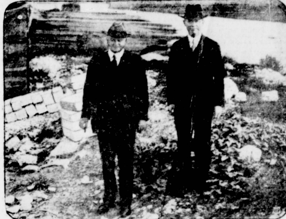
President-Elect Hoover at Miami and Gov. Doyle Carleton of Florida looking over the reconstruction work in South Bay, Fla., one of the sections laid waste by the devastating floods of Lake Okeechobee.
