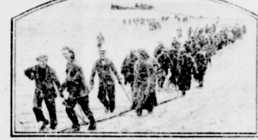
Landing the cable—one of the most dramatic moments in the job of establishing cable communication between continents. This scene is duplicated at both ends of the operation—first when the shore end is landed at the beginning, and again when the task is successfully completed.
