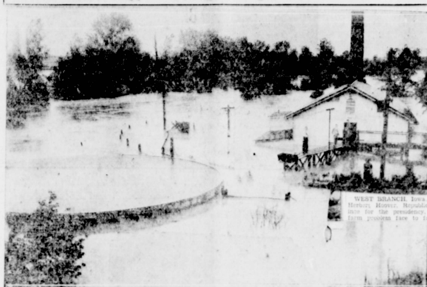
Milledgeville was one of the cities hardest hit by the storm and flood, which swept Central and South Georgia last week. Photo shows water up about Milledgeville water plant. Sluiceway Creek swept over its banks and dashed the depth of the waters may be gathered from the fact that the reservoir shown in the photo, stands 17 feet above ground. Water picture was made water was within four feet of reservoir top.
