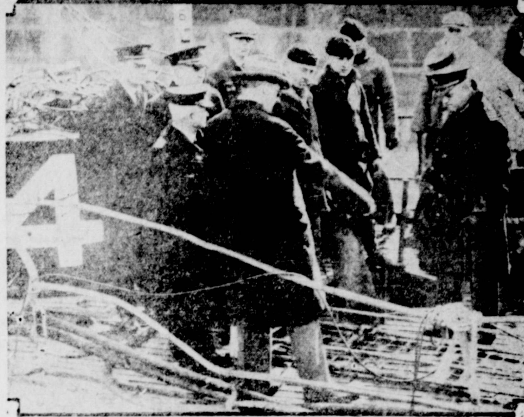
Secretary of Navy Wilbur looks down through the hatchway at the damage done in the forward compartment of the ill-fated S-4 while she is in dry dock at the Charlestown Navy Yard, Boston, Mass. (International Newsreel)
