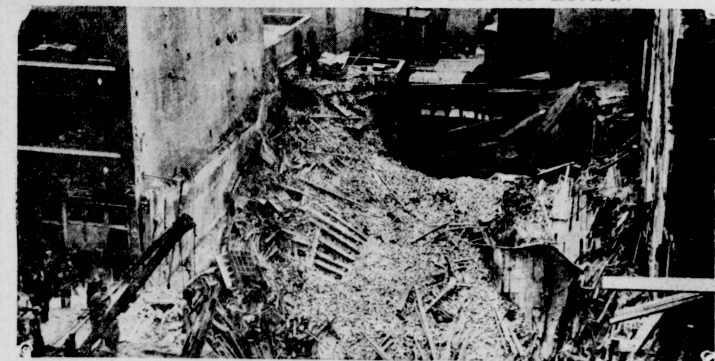
Workers are combing through the ruins of two three-story buildings that crashed with a thundering roar into a New York city subway excavation, seeking the bodies of other victims of the accident, in which it is known that two men were killed outright.
