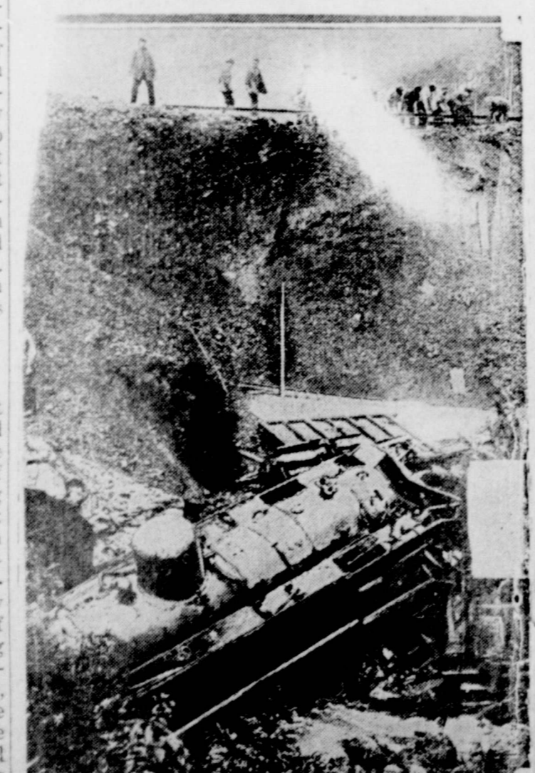
Here is one consequence of the disastrous floods now raging in Germany. High waters undermined railroad tracks at Wernigerode, causing a passenger train to plunge over an embankment. Nine were killed and twenty-two injured. Photo shows the wrecked train. (International Review.)
