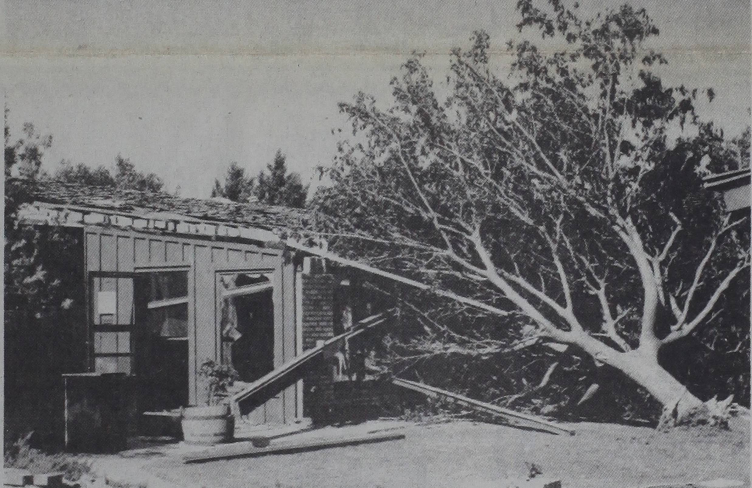
TORNADO DAMAGE.... The J.D. Cage home just east of Muleshoe was virtually destroyed last Saturday by a funnel cloud. The large tree at the right was uprooted, and is thought to be the one that witnesses said was lifted 100-150 feet into the air by the funnel, before being dropped back to earth.
