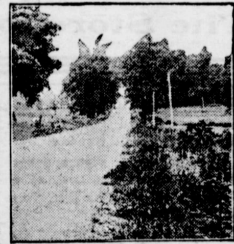
Bituminous Macadam Road.
