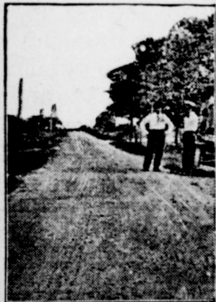
Soil Road in North Carolina.
