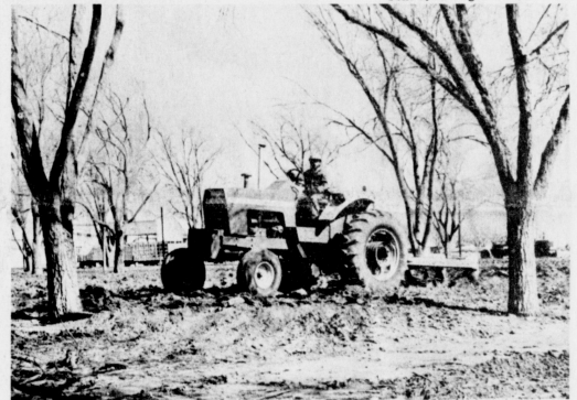
PARK IMPROVEMENT.....Work continues levelling and plowing the local park to be ready for the spring-summer season. Here Muleshoe Ford Tractor Company equipment plows the land for planting.
