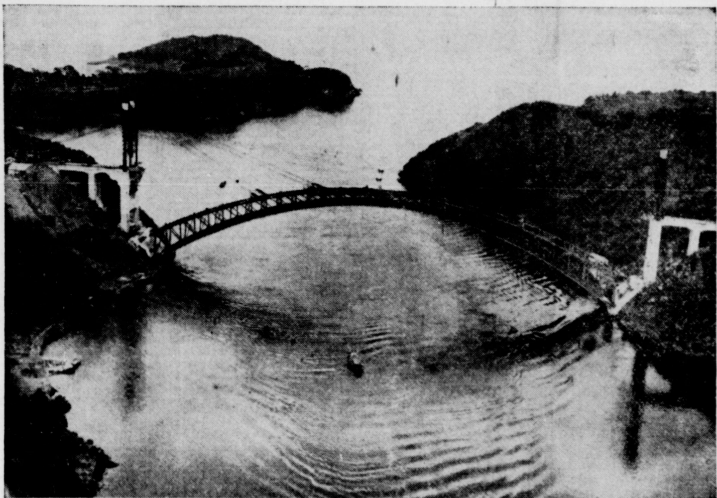
ARCH IN THE EAST—A new single-span steel arch bridge now links Nagasaki with Sasebo, on Kyushu Island, and marks the completion of the third largest bridge of its kind in the world. It was built at a cost of about $1,500,000, is 712 feet high at the center and 1042 feet long, a thing of beauty and one of Japan's prides.
