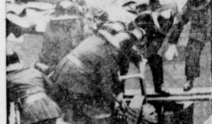
THERE'S NO END TO IT—Although Hitler's World War II Luftwaffe doesn't fly over London any more, it is still taking a toll. When Frank Moran, a workman, fell into an old bomb crater, firemen had to be called to help extricate him. A new building is being erected on the site.
