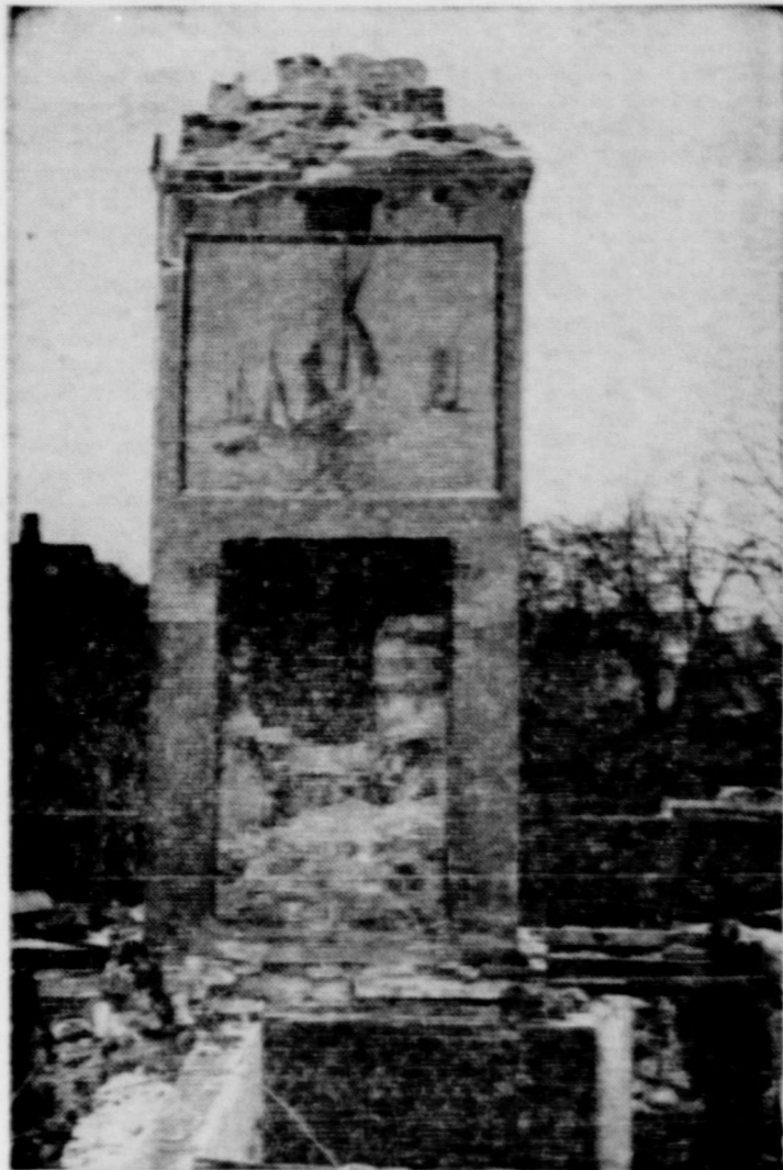
THE LAST TO GO —When a former snowplace was being torn down in Elizabeth, N. J., a delicate mural atop a dining room fireplace was the last remnant of elegance. Built in 1870, the mansion was sold to an auto dealer firm by the last of a succession of owners in 1951. Vandals took over and reduced its one-time elegance to an eyecore and the firm was ordered to board the mansion up, repair it or tear it down.
