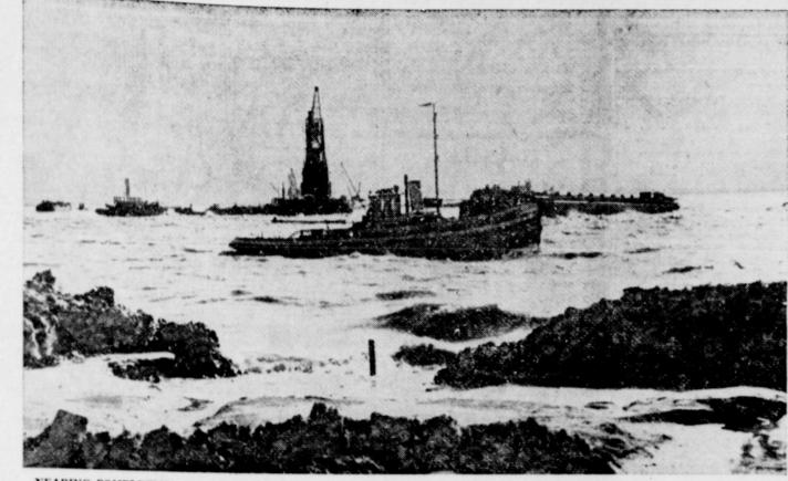
NEARING COMPLETION-A small muddy gap is all that remains to be filled by engineers in a project to restore farmland from the Zuider Zee. Begun in 1951, the program was set back by disastrous floods in 1953, when workers were diverted towards stricken islands in Holland's low country. An 18-mile dike will make the country safer from watery invasions.
