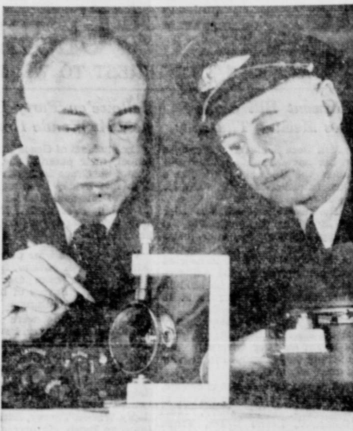
IT'S NEW—The gyroscope heart of a revolutionary new steering and direction-finding system is being explained in New York by Clark Smith, left, Bendix Aviation Corporation technician, to navigator Mauritz Sundt of the Scandinavian Airlines System. Designed for flights over the polar regions where magnetic compasses go haywire, it spins 22,000 times a minute, and automatically solves direction problems.
