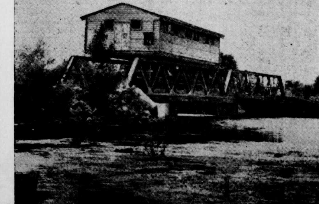
OPTICAL ILLUSION —This is not an old covered bridge, as it appears; actually, it's a large barrack building being moved over a bridge at Goose Island, Wis., to a new location as headquarters for a wild game club. Too wide for the bridge, it had to be hoisted over.
