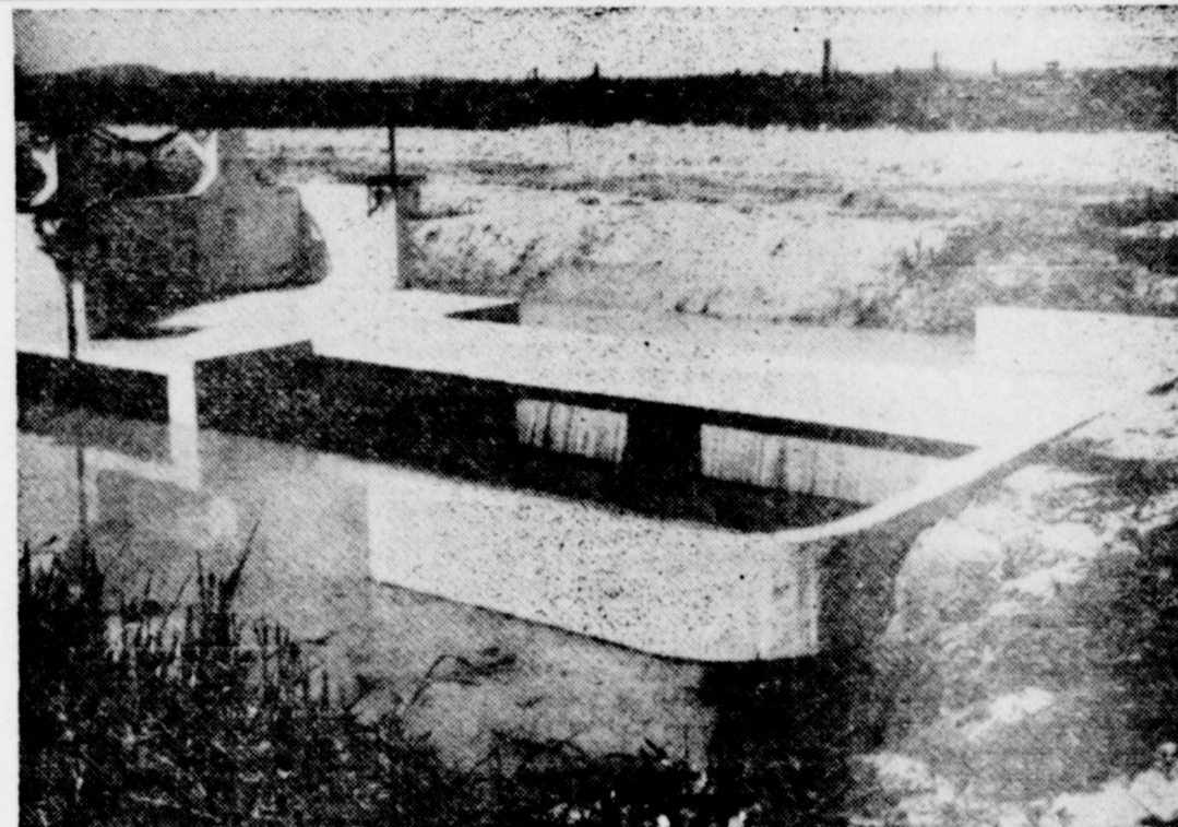
CULTIVATING THE LAND—This control lock is part of an extensive irrigation system being constructed by the Perak State Government of Malaya in Changkat Jong area. A five-year plan in progress is expected to turn 6000 acres of wasteland into rice paddies for Chinese colonists who have agreed to keep the land under cultivation.
