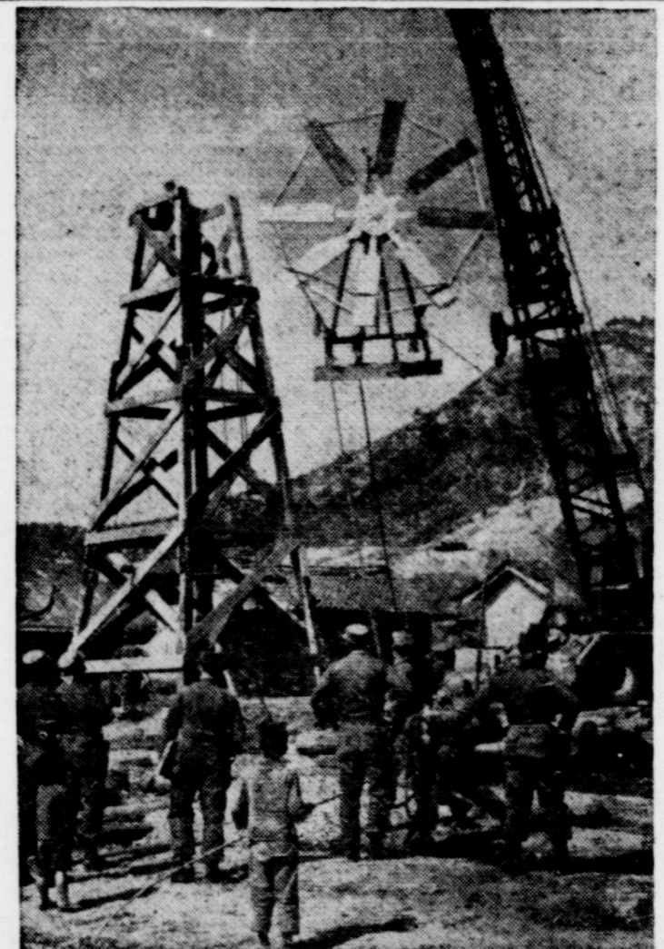
OPERATION WINDMILL — Members of the 3rd Engineer Combat Battalion watch anxiously as a crane carefully swings the upper assembly of Korea's first windmill into position. Intended to test the practicability of pumping water by wind-power, the mill is located in a recently resettled village north of the 38th parallel. If it works, the natives will benefit.
