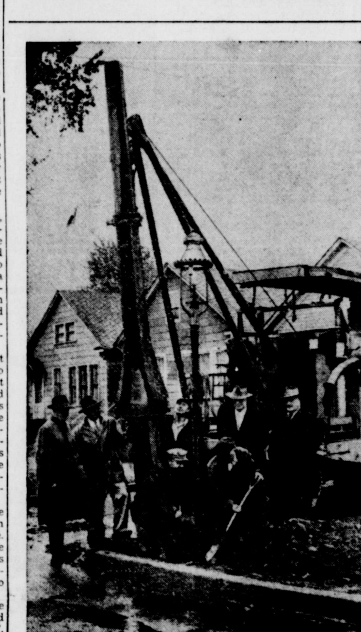
IT'S THE END!—Snuffing out the last flickering holdover of the gaslight era in Chicago, city workmen are watched by gas officials as they remove one of the last 18 gas street lights in the Windy City. Installed in the "nineties," the lights gave off only one-twentieth of the glow of their new electric replacements. Residents nearby will have to learn to live with all the unfamiliar night-time light they'll be getting.
