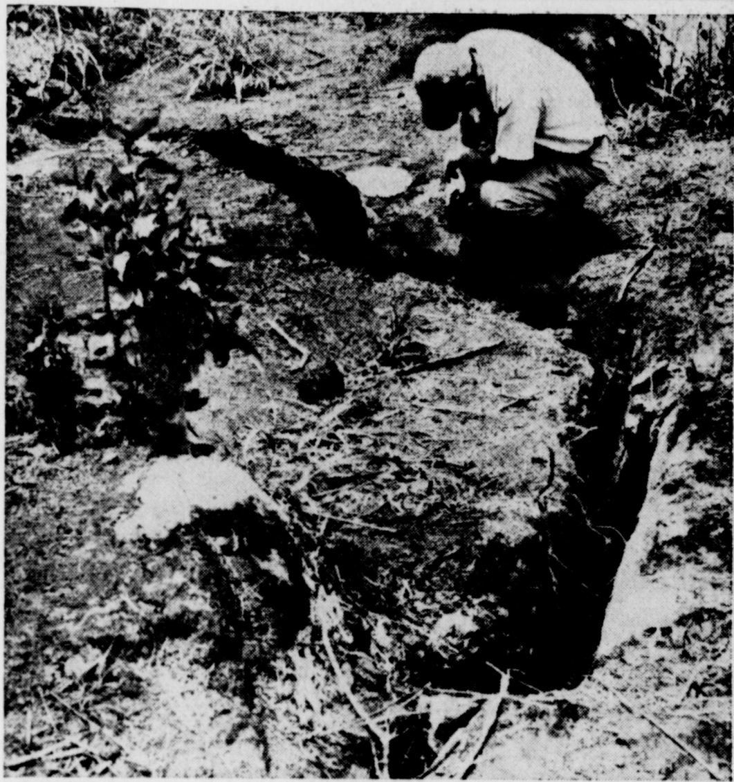
THREAT IN PANAMA —A surveyor is checking a deep crack which threatens to open wider and cause a landslide which might block the Panama Canal. The 600-foot-deep crack is in a rock ledge overlooking the canal in the famed Gaillard Cut. First noticed some years ago, the crack has been widening recently and the rainy season could create a real avalanche.
