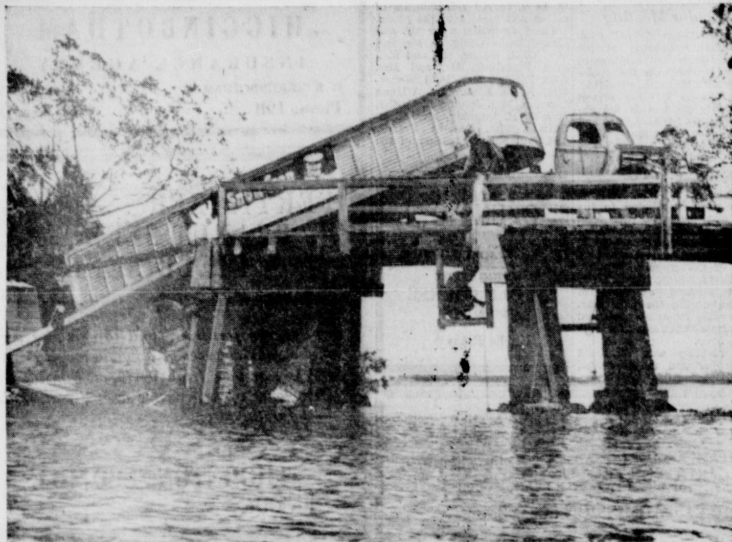
DELAYED CARGO —Production at a Florida orange concentrate plant was considerably slowed when this trailer-truck's cargo of fresh oranges failed to arrive on schedule. The truck's rear wheels smashed through the wooden planking of this bayou bridge at Bradenton. It took workmen all day to transfer the fruit to another vehicle and get the load to the plant.
