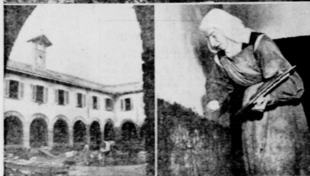
NUNS BUILD OWN CONVENT—Working from plans drawn by hired architects, these Carmelite nuns are building their own convent near Turin, Italy. Four of the 13 who will live there are shown in top photo carrying heavy cement bases. The sisters took lessons from two months and did all the work with some volunteer help, lower left. Sister Theresa is shown at right handling the tools of a mason's trade. The nuns will live in cloistered silence in the sisters order.
