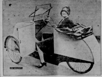
A woman rider starting out in a portable collapsible cycle car with a three-speed gear and a front brake, a recent innovation in London, the popularity of which is increased by the fact that it is taxless.
