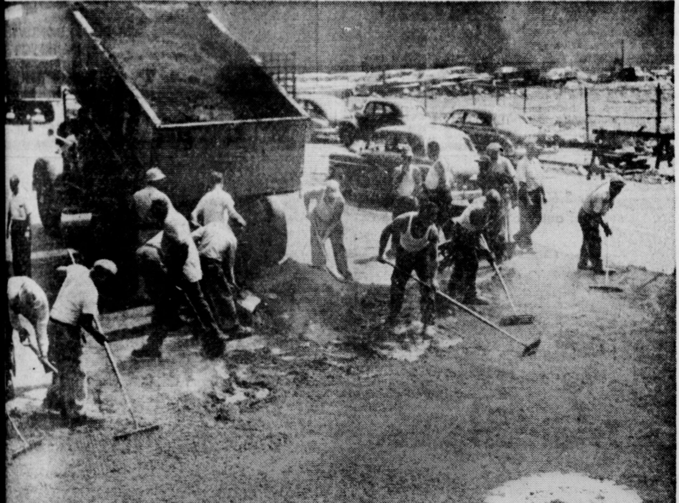
LAUNDRY TRY-OUT —A crew of workmen are paving a section of a New York avenue with rubber. The rubber is mixed with asphalt, a conventional paving material, and it is believed the new blend will add resiliency to lengthen the life of the street. The rubber may also act as a sound-deadener when heavy trucks roll over the new paving composition.
