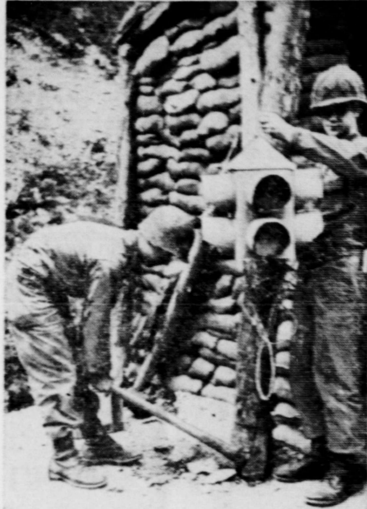
CANNED SAFETY —Augmenting safety measures along heavily-traveled UN supply routes near the Korean front, a modern-type traffic signal is trimmed into shape by two members of the 45th Infantry "Thunderbird" Division. The three-way light was made from food and coffee cans and gets its illumination from Christmas tree bulbs. Cpl. Irving J. Laborovitch, left, of Minneapolis, and Pfc. John Stunglen, Philadelphia, are setting it up.
