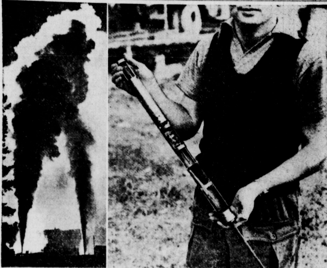
ONE OF NATURE'S WONDERS—In New Zealand, where the cost of hydroelectric power is high, scientists are seeking economical methods by tapping pockets of underground steam and harnessing the power. Two new steam bores in the Wairakei area are shown at left. The roar of escaping steam is almost deafening and giant mufflers, such as the one shown at right, are placed on each test bore to lessen the sound by allowing steam to expand before it escapes.
