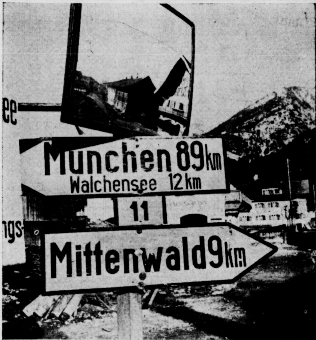
NOTE TO CHAMBERS OF COMMERCE—What appears to be a promotion picture of a Bavarian village in Krueen, Germany, is actually a safety device for drivers—placed on top of a road sign. It's really a mirror that reflects oncoming traffic around a corner.
