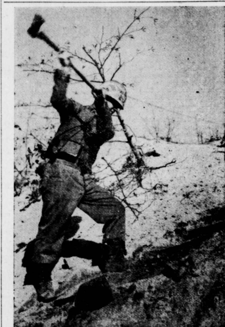
BUILDING UP TO SOMETHING—Marine Pfc. Tony Melim, of Lowell, Mass., is just trying to make life and fighting conditions more tolerable in Korea. He's chopping away at that hard-packed earth in an effort to build a series of steps to his bunker. Melim knows only too well that there's nothing like the comforts of home, even if "home" right now is on the front lines.
