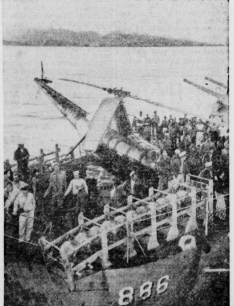
UNUSUAL LANDING—A helicopter from the cruiser USS Los Angeles looks out of place among the depth charge racks and depth charges on the destroyer USS Orleck, in Far Eastern waters. Suffering power failure during a routine mid-air transfer of personnel from one ship to the other, the 'copter was skillfully slipped onto the fantail, just missing the after five-inch gun mount. (U. S. Navy Photo)
