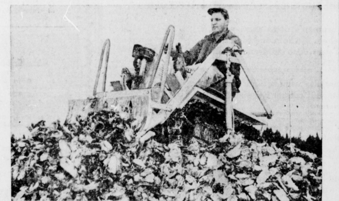
EVERY LITTLE BIT HELPS—Oyster shells are being used in Olympia, Wash., to help reclaim the gooey tidelands in the area. Bob Bower is shown operating a tractor at low tide in Mud Bay, compressing the shells into the soft ground to form a firm base.
