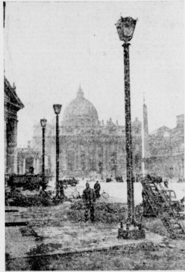
NEW LIGHTS IN OLD CITY —Cast iron lamp posts have been added to Piazza Pio XII, facing famous St. Peter's Square in Rome, Italy. After the old Borgo quarter had been demolished and new Vatican palaces built in front of the Basilica on the opposite side of the square, some lights were needed to complete the effect. The new posts, with their old-fashioned cast iron
