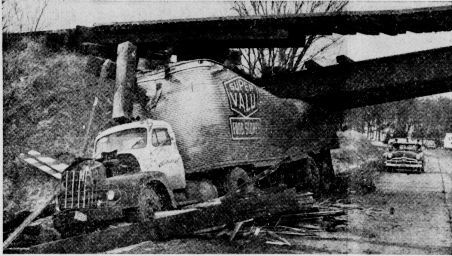
BAD LUCK DOGGED HIM —Because he tried to avoid a reckless auto driver approaching on the wrong side of the road, Israel Scherbenske crashed his trailer into a railroad bridge in Minneapolis, causing huge beams and timbers to topple down. The trailer was crushed as timbers ripped the front and hood of the cab without entering it, and Scherbenske was lucky to be alive.
