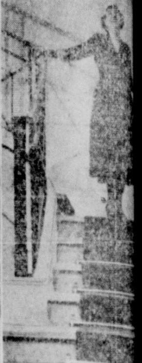
AT HOME ABROAD —The General's wife stands on the main staircase of the villa Marnes-La-Coquette. The simple design of the wrought-iron bannister gives some indication of the unaffected decor of the gracious home, which the man, with the weight of the defense of Europe on his shoulders, is apt to relax. The secluded villa is not far from the General's SHAPE headquarters.
