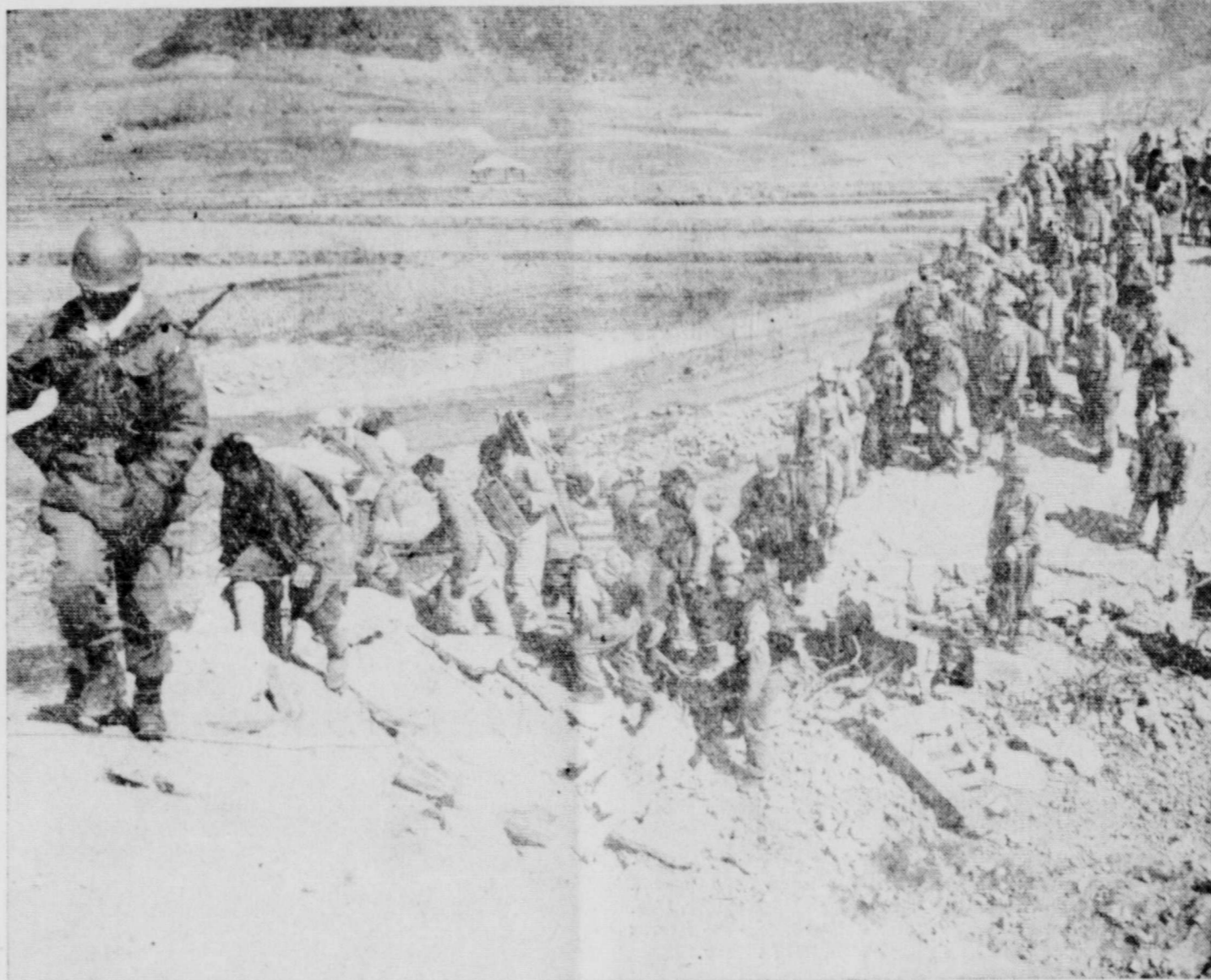
ROKS AND RUBELF—Republic of Korea troops slow down for rubble climbing as they go up and over a ruined bridge during the advance against massing Communist forces. In contrast to the shattered concrete, a flimsy, wooden-poled structure with roof of straw still stands intact in the center background. (Acme Photo by Bert Ashworth, Staff Photographer.)
