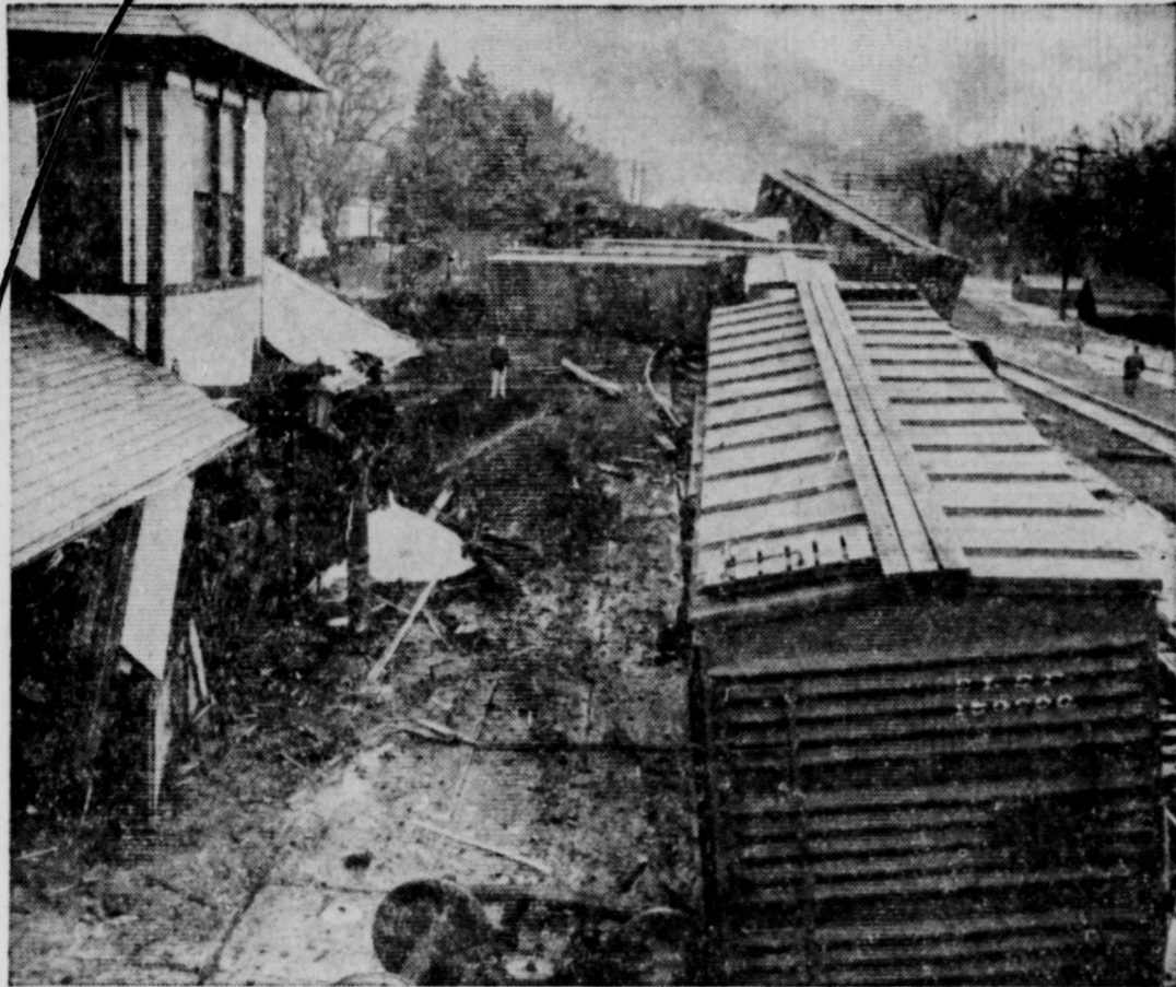
MIXUP —When 27 cars of a 140-car freight train were derailed, one smashed into the station at Tuxedo Park, N.Y., wrecking part of the 65-year-old building. The heavily loaded train was en route to Jersey City from Buffalo, but there were no injuries in the early-morning accident.
