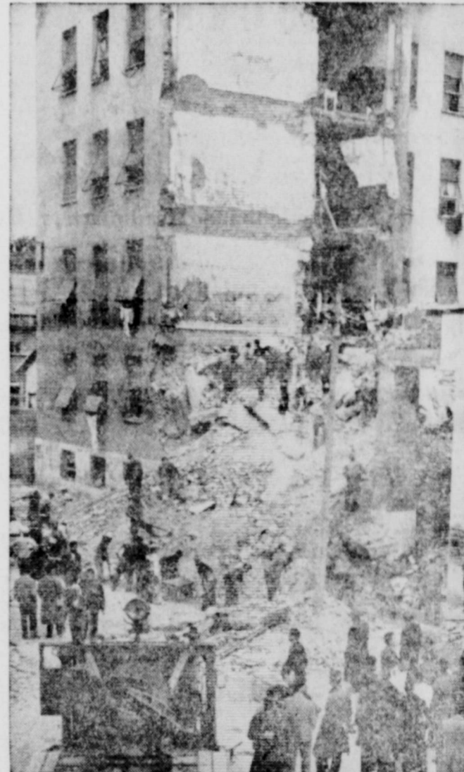
UNCERTAIN LIVING —After a section of this building collapsed, killing three persons and injuring 12 in Rome, Italy, workers began clearing the rubble and masonry. Formerly a school, building has recently been occupied by refugees. The cause of the unexpected collapse has not been found, and the city's Mayor was threatened by an angry crowd when he visited the scene.
