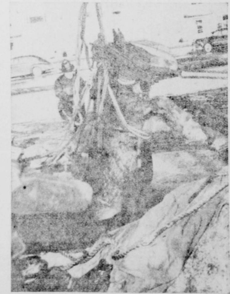
UP HE GOES! —This horse fell into a hole near a construction job where he was pulling a sidewalk plow in Milwaukee, Wis. It took a block and tackle, set up by firemen, and a lot of time to get the animal out of it, but he seemed to understand the trouble and cooperated by not being too vigorous.
