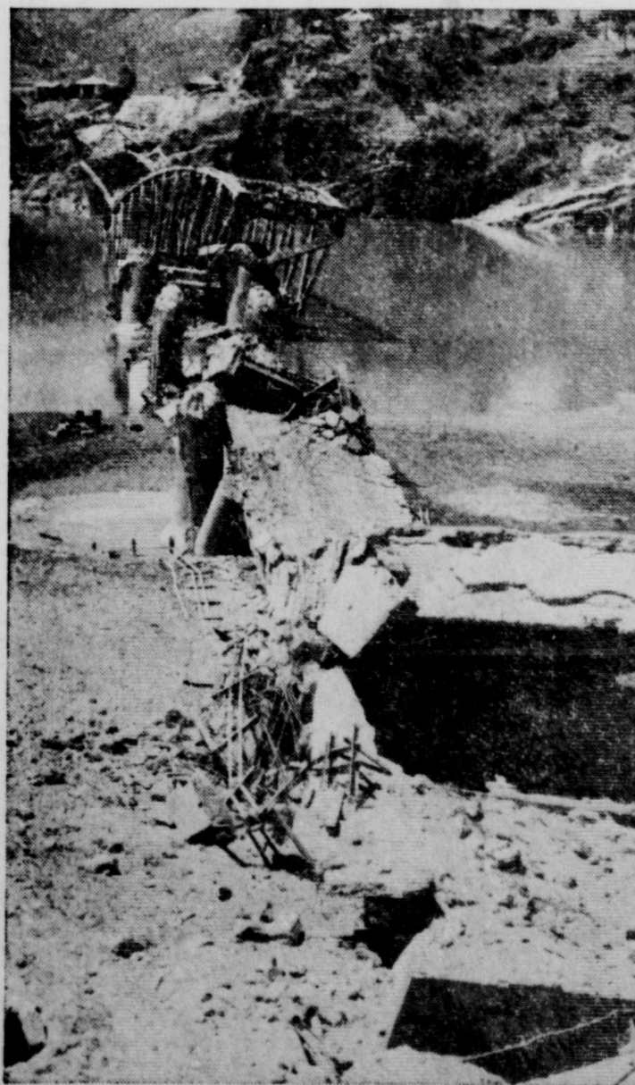
NO ENTRY—Red hordes won't cross the Nakdong River into territory still held by United Nations forces in Korea on this bridge. American demolition experts placed explosive charges at various points of the bridge and its approaches and blew it to pieces.
