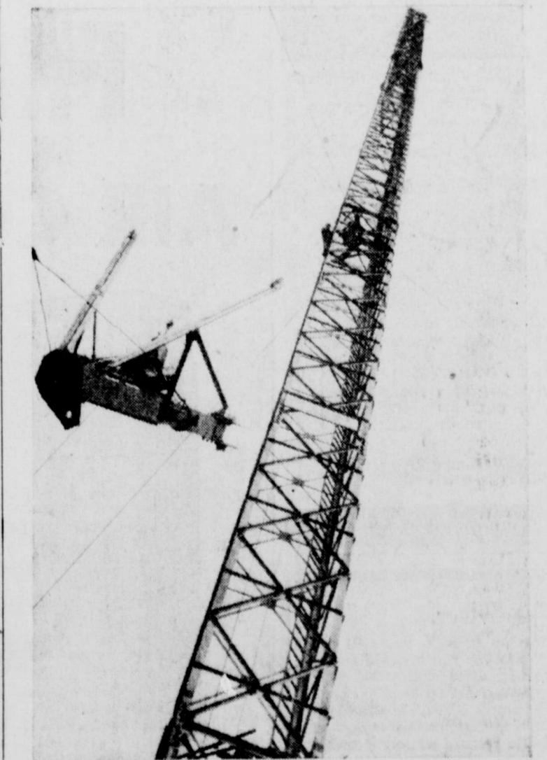
U. S. TRANSMITTER IN BERLIN —This high frequency radio transmitter, capable of insuring the flow of U. S. Army communications in case of another blockade of the German city, has just been put into operation. The tall, slender steel tower rises some 320 feet above the compound of Army Headquarters in Berlin.
