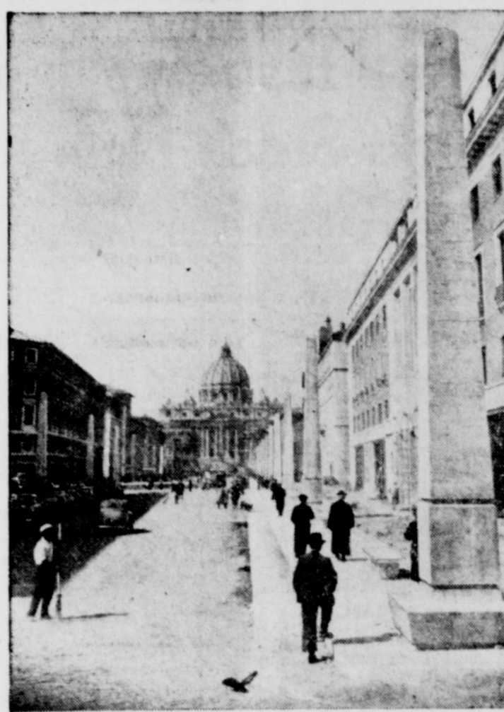
LINING THE WAY —A Holy Year addition on the Via Conciliazione, main approach to St. Peter's Basilica, in Rome, are the new white carrara marble obelisks erected by Vatican engineers. Marble benches on which weary pilgrims may rest on their way to the church have been placed between the 25-foot-high columns.
