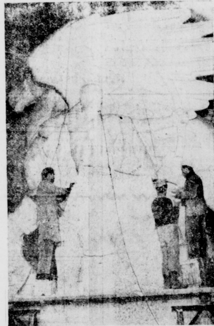
DESTINED FOR U.S. —Workmen apply a preliminary clay coating to a 20-foot-high chalk model in a bronze works in Rome, Italy. The statue, one of four executed in America, will be cast in bronze as a gift from the Italian Government for installation on the Arlington Bridge in Washington, D.C.
