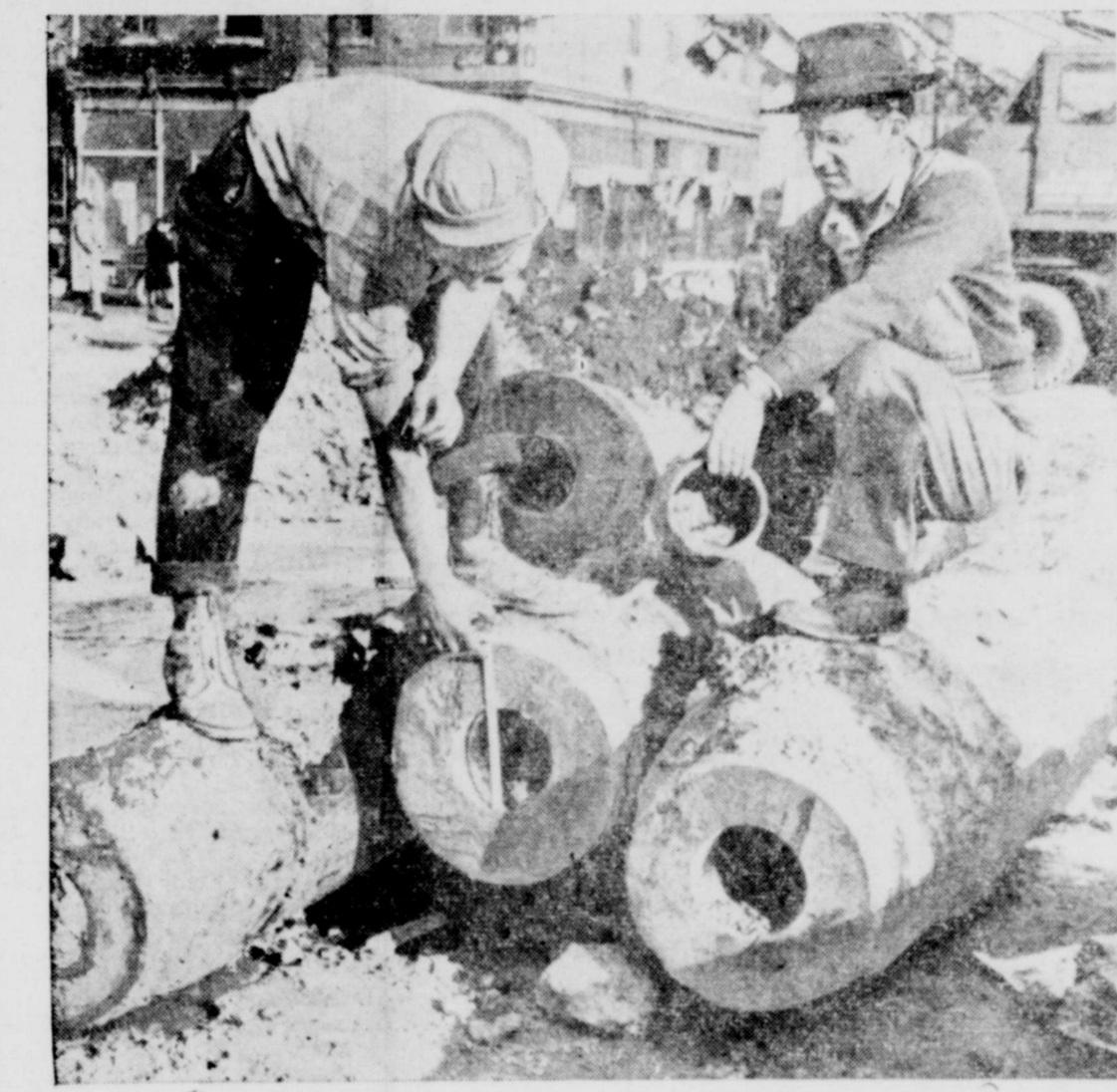
AWAY WITH THE OLD—Hollowed-out tree trunks that brought water to the city, from the eighteenth century until present times, are examined by workmen in Philadelphia, Pa. This antiquated system was old when most of the country was drinking well water. Al Tyman, right, holds one of the cast iron pipes used as a connecting link between logs as Frank De Felippes, foreman of the construction crew, estimates the capacity of the units.
