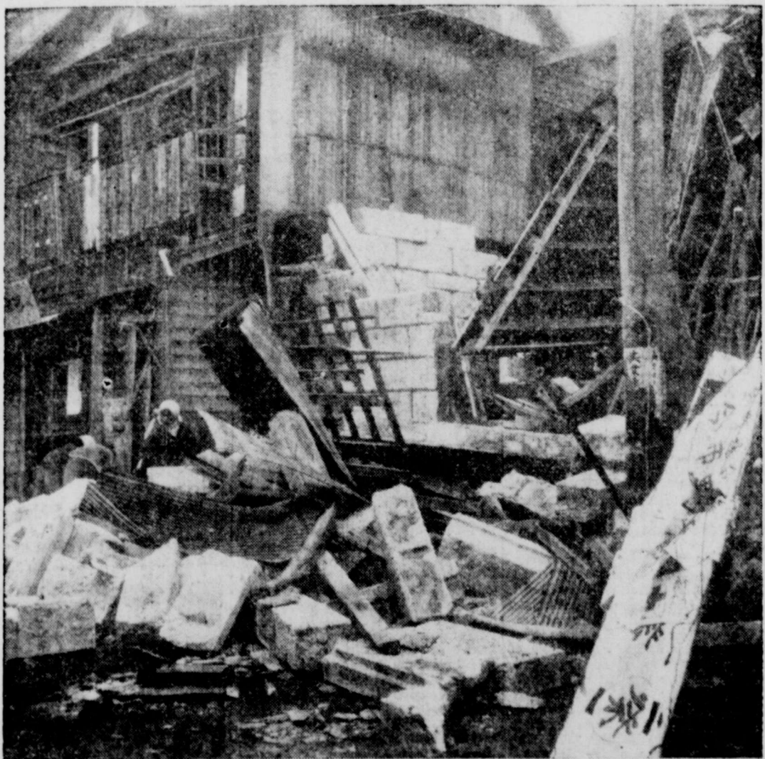
HARD HIT —The worst earthquake Japan has experienced since the Tokyo disaster of 1923 has now destroyed 874 houses. More than 5000 other houses were partially damaged by the wave of three quakes. Hardest hit was the town of Imaichi where 80 per cent of the dwellings suffered damage, and stone houses like the one shown here were demolished.
