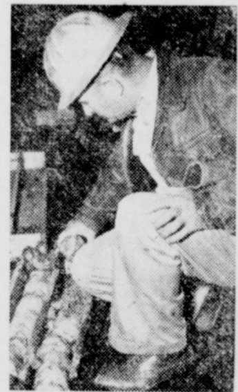
LONE STAR GEOLOGIST saves "core" from well being drilled for further study. "Core" reveals information vital to proper completion and operation of wells. This picture was taken on the rig at right, the night the well was successfully completed.
